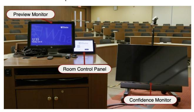
Walking into a classroom you'll see two displays on top of the classroom lectern: the Preview Monitor for the classroom computer and the Room Control Panel (the smaller of the two displays). You'll also notice the Confidence Monitor, with attached camera, on the floor set at an angle for you to see as you lecture.
